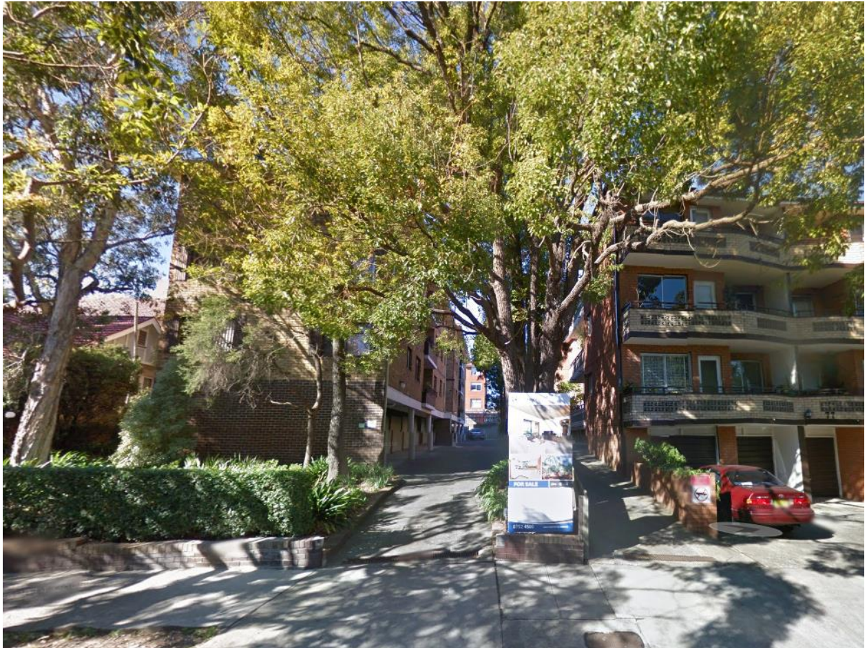
Fig. 6 – Photograph of the RFB to the south-west (75 The Boulevard, Dulwich Hill)
