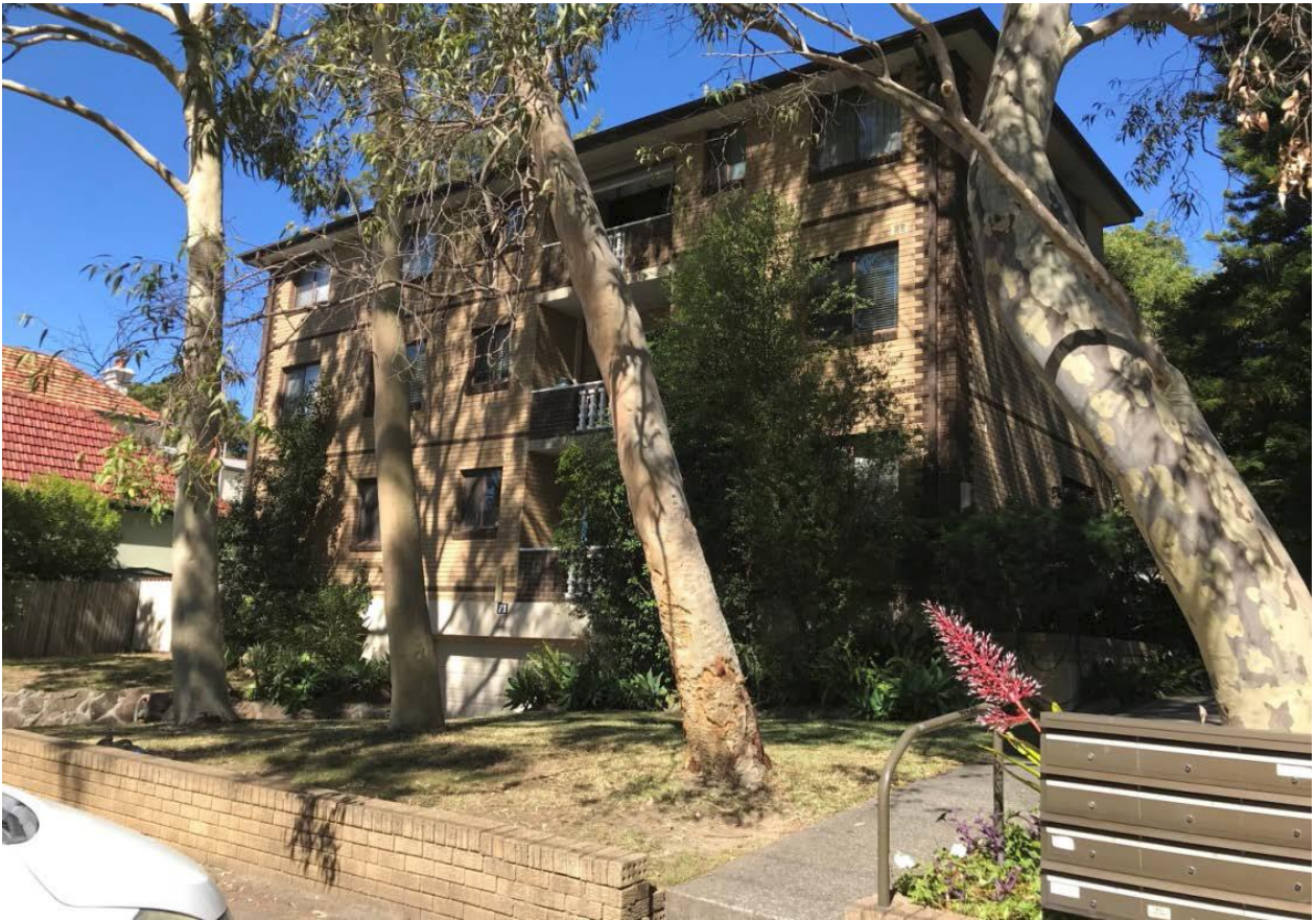
Fig. 5 – Photograph of the RFB to the north-east (71 The Boulevard, Dulwich Hill)
